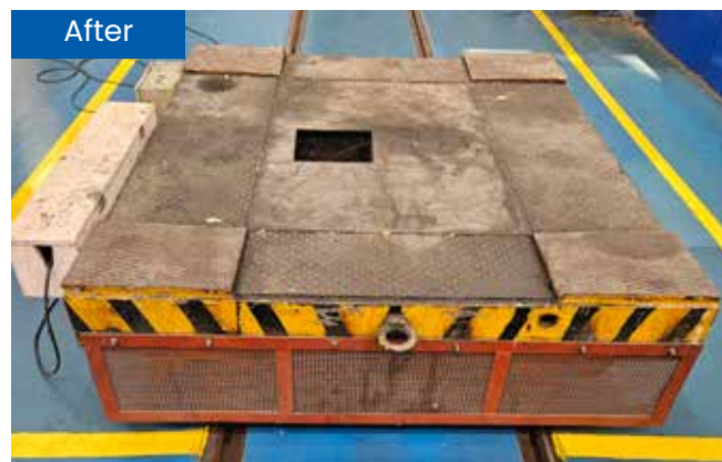
A trolley wheel guard was installed in the trolley to eliminate leg injury and minimize the risk during operation.
