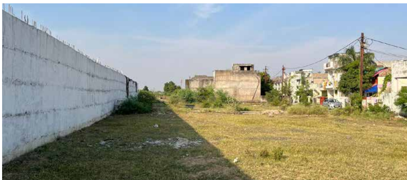
A View of the 12 Feet Reinforced Cement Concrete (RCC) Curtain Wall for Flood Control at Mandideepat Mandideep
