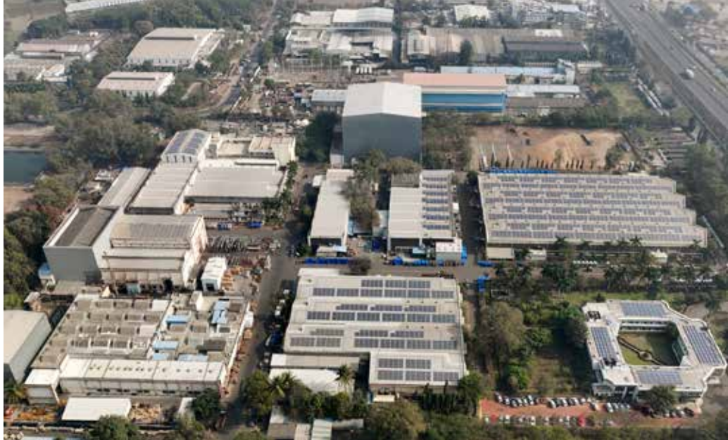
Switchgear Products Manufacturing Unit at Nashik, Maharashtra
