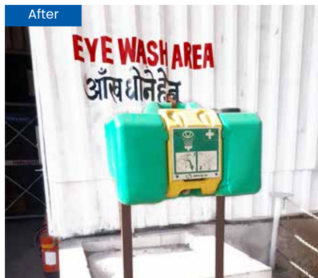
Portable eyewash was secured and it is easy to carry across locations. In addition, no maintenance is required for the same.
